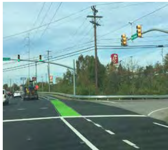
The bike lane along Old Hickory Blvd extends through the intersection and green pavement markings highlight the potential conflict area.
