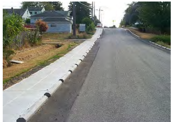
Seattle has developed a low-cost sidewalk program that uses lower cost materials, such as stamped and stained asphalt, to reduce construction costs. Seattle is also proposing new public-private partnerships to expand the sidewalk network.
