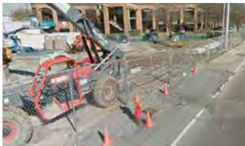
Lack of pedestrian accommodations during construction along Hillsboro Pike
