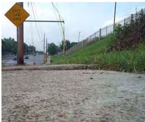
Horizontal cracks in sidewalks create tripping hazards.
